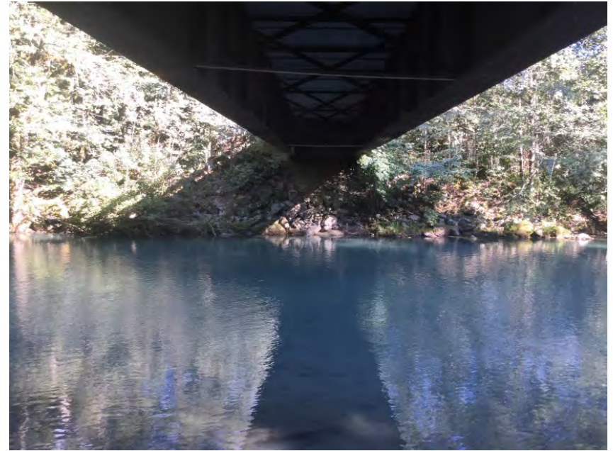
Left Bank Abutment
