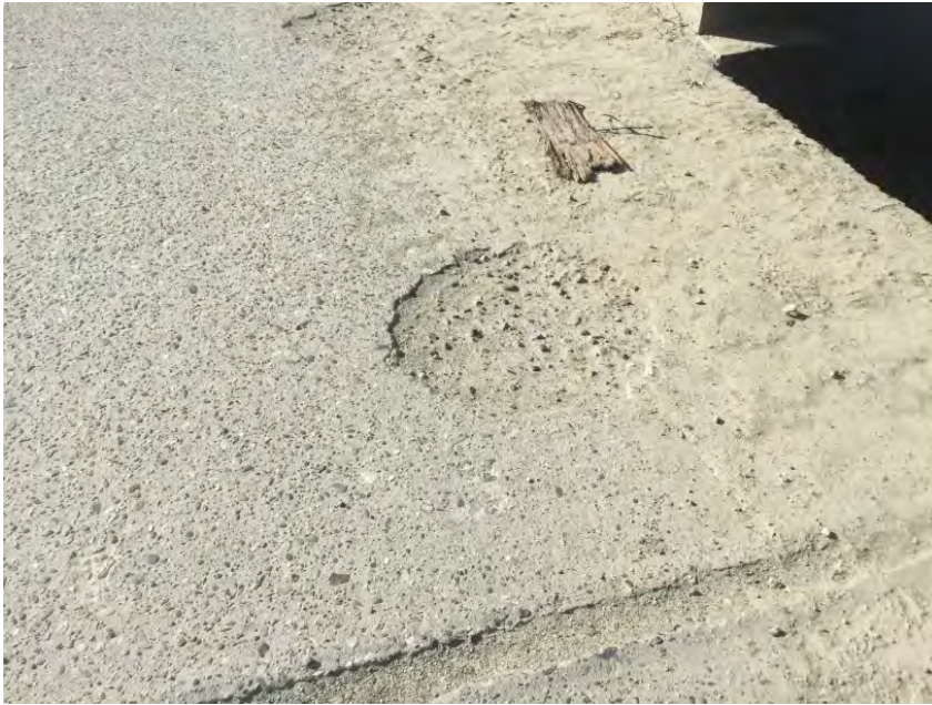
Typical Grout Pocket Condition
