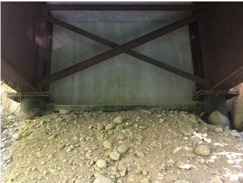
Left Bank Abutment
