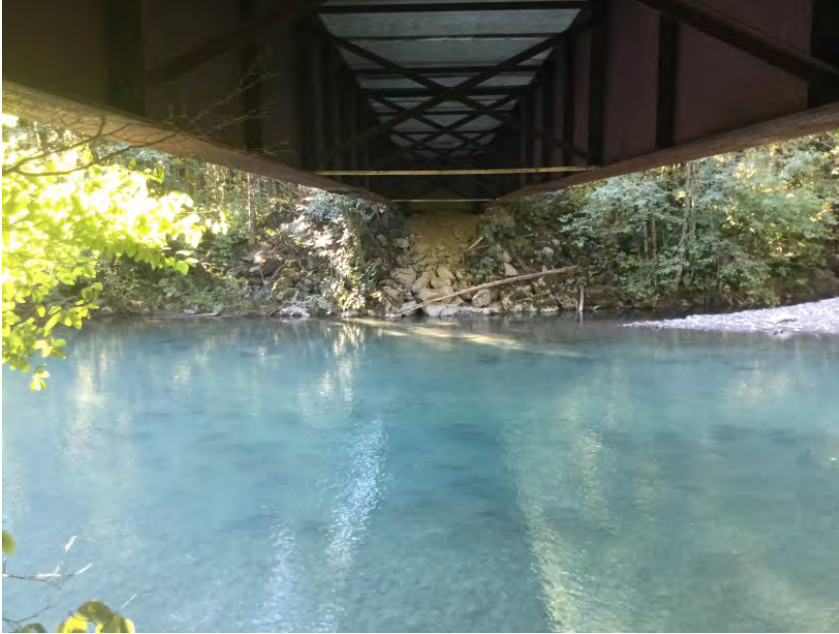
Right Bank Abutment
