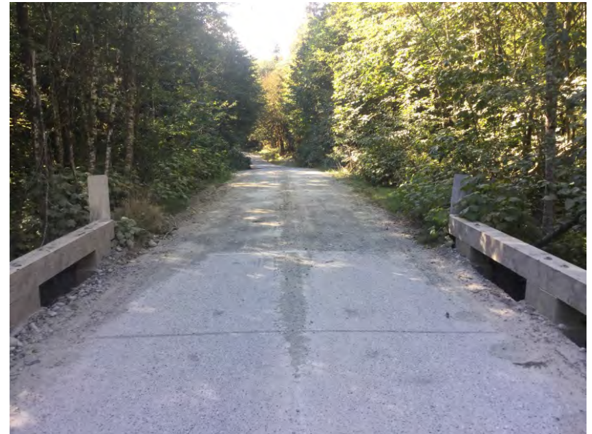
Right Approach Facing Away From Bridge
