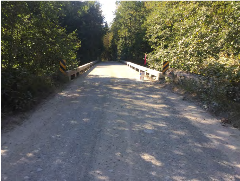
Left Approach Facing Bridge
