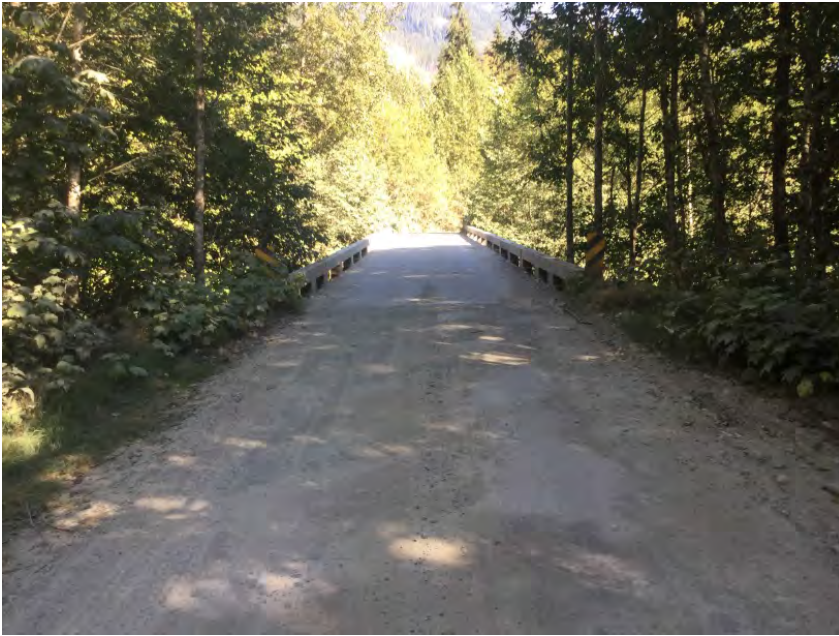
Right Approach Facing Bridge
