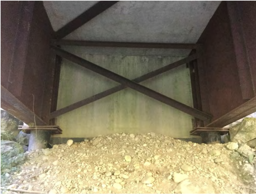
Right Bank Abutment
